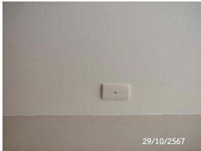
Fire Alarm Indicator Lamp
