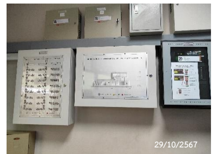
Graphic Annunciator Fire Alarm System
