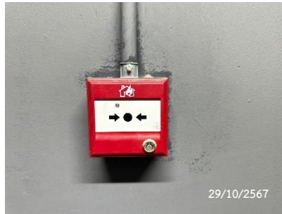
Fire Alarm Manual Call Point
